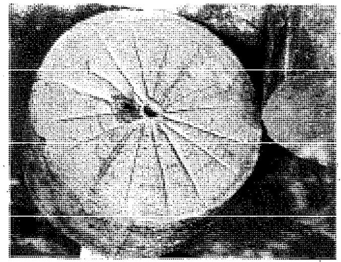
Marks like this are made in both faces with the corner of a small board. On the second day you can fit them together and turn the top enough to seat them nicely. The concrete will be well cured in 3 to 4 weeks.
