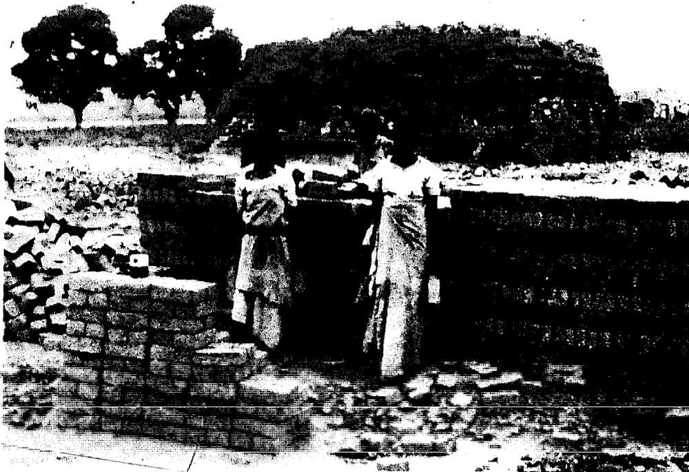
Wood-fired clamp under construction by lady brickmakers. Lack of suitable hand trucks leads to excessive carrying. Some shape defects can be seen in bricks in the foreground
