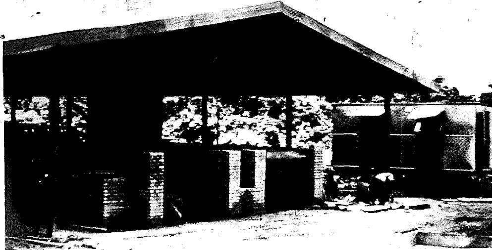
An originally constructed, side-fired double chamber kiln specially designed for wood firing, in use at Asokwa and Ankaful brickworks. Fuel consumption was high because the kiln is intermittent and no heat is re-used from the bricks cooling down from previous fire. Subsequent measures applied to increase the height of the side walls are understood to have improved efficiency
