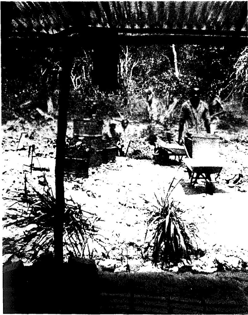
Improvised water transporting system with tub carried in wheel barrow – water supply is nearly ½ km away
