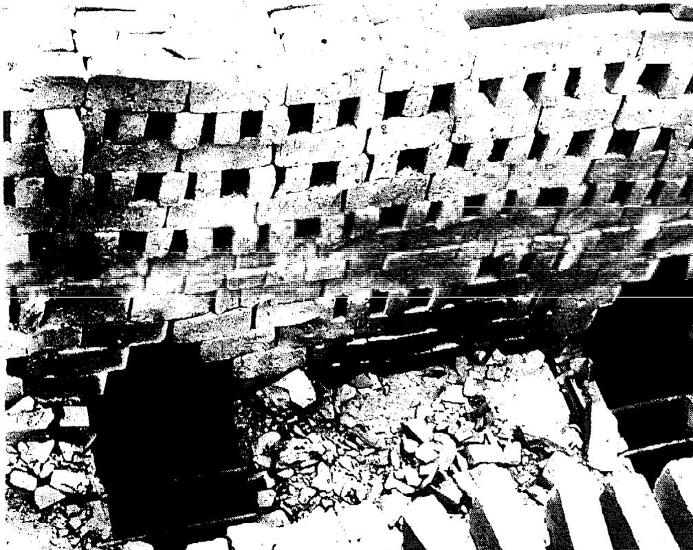
Firing channels act as hearth under setting, often producing more consistent results than large "tunnels" through the brick setting itself
