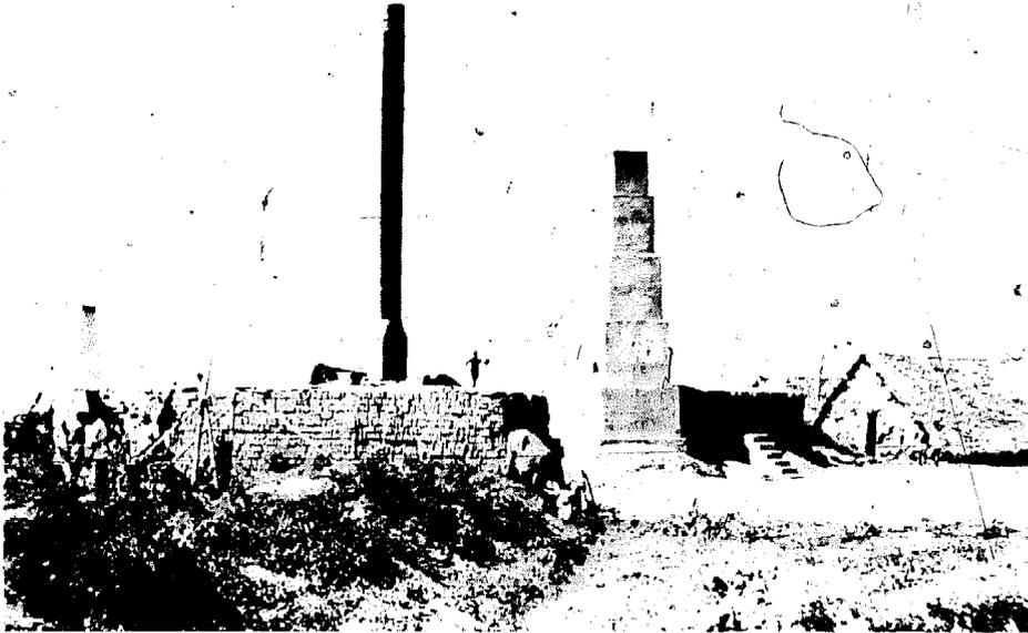
General view of plant showing movable metal chimney alongside permanent brick chimney.
