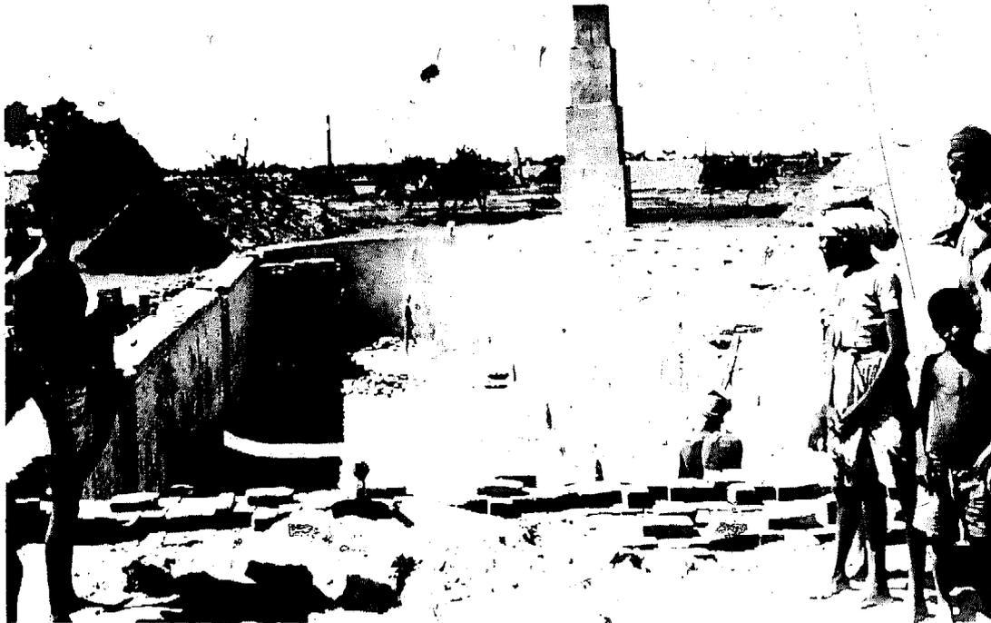
Vacant chambers of Bull's Trench kiln taken from the point where the dry bricks are being set, looking
