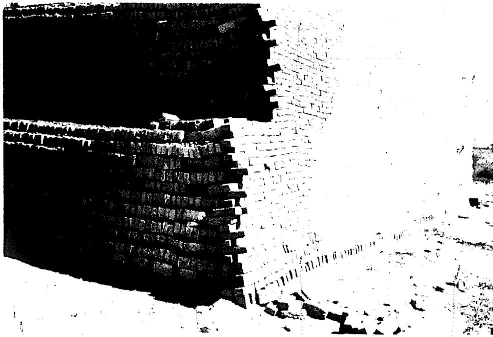
Extremely high standard of coal fired clamp construction likely to achieve a high efficiency of fuel consumption and consistent burning
