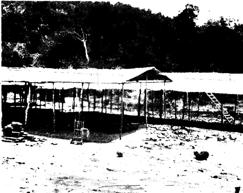
Corrugated-iron roofed working and drying sheds constructed out of rough timber cut from adjacent forest. Buildings need provision to adjust for different ambient drying conditions
