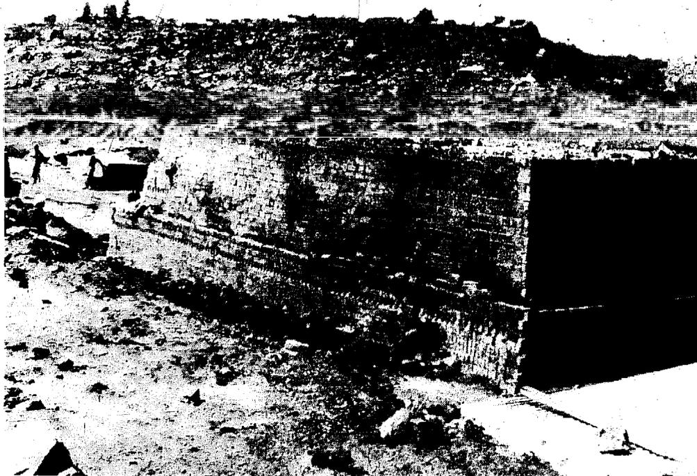
Large scale clamp fired with coal and clinker waste from power stations
