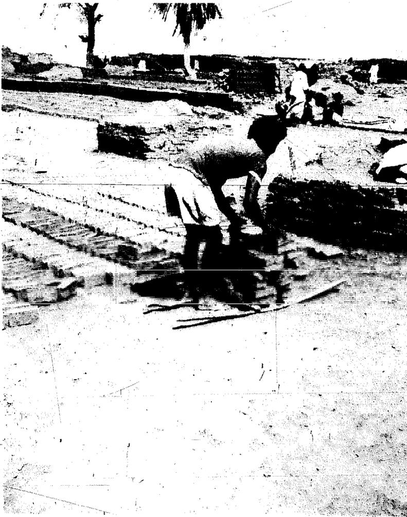
When fully dry, loads of 50 bricks stacked on carrying litter
