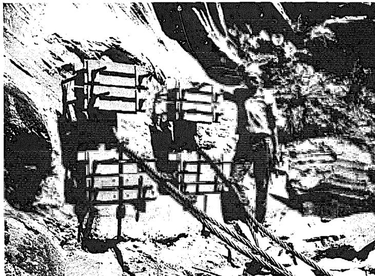
Rock anchors used for main cable anchorage
