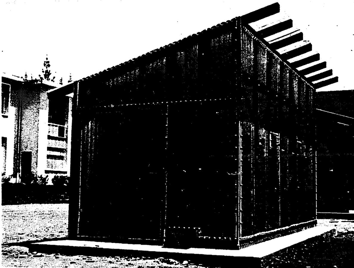
Figure 1. General View of the Lumber Dryer. The Inlet Vents can be seen on the Right, and Outlet Vents on the Left.
