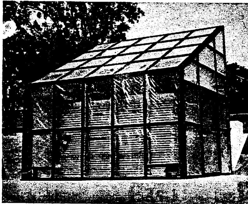
Figure 1. Solar Kiln, Recirculating System with Partial Air Venting. Sheet Reflectors Partially Visible on the East and West Sides.
